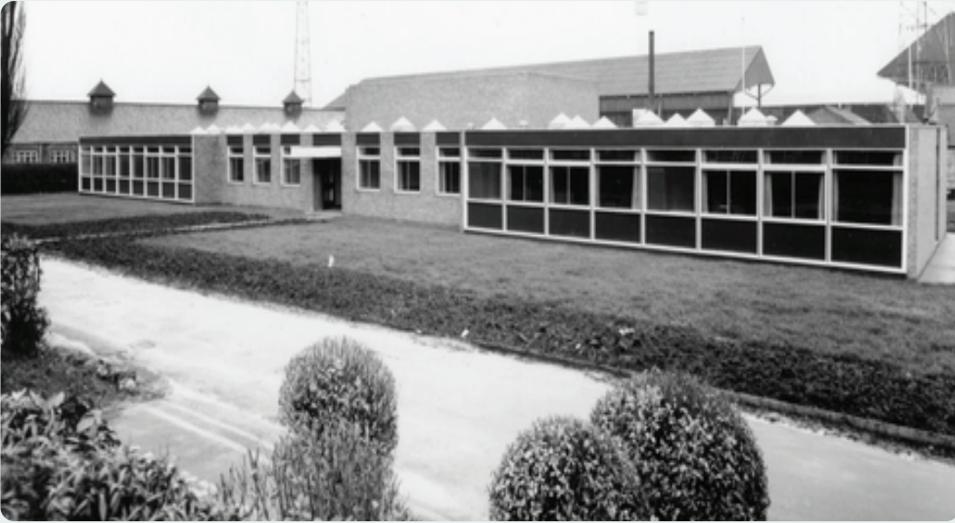
Figure 2: Middlesbrough General Hospital
